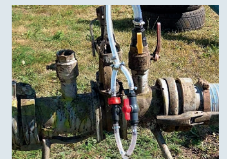
Addition via suction hose
